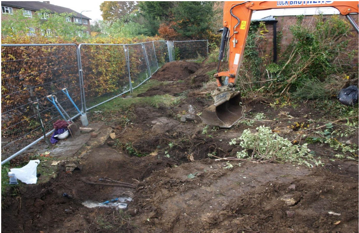
Plate 9: Showing eastern end of evaluation Trench 3, live water-main visible in foreground, viewed from the east
